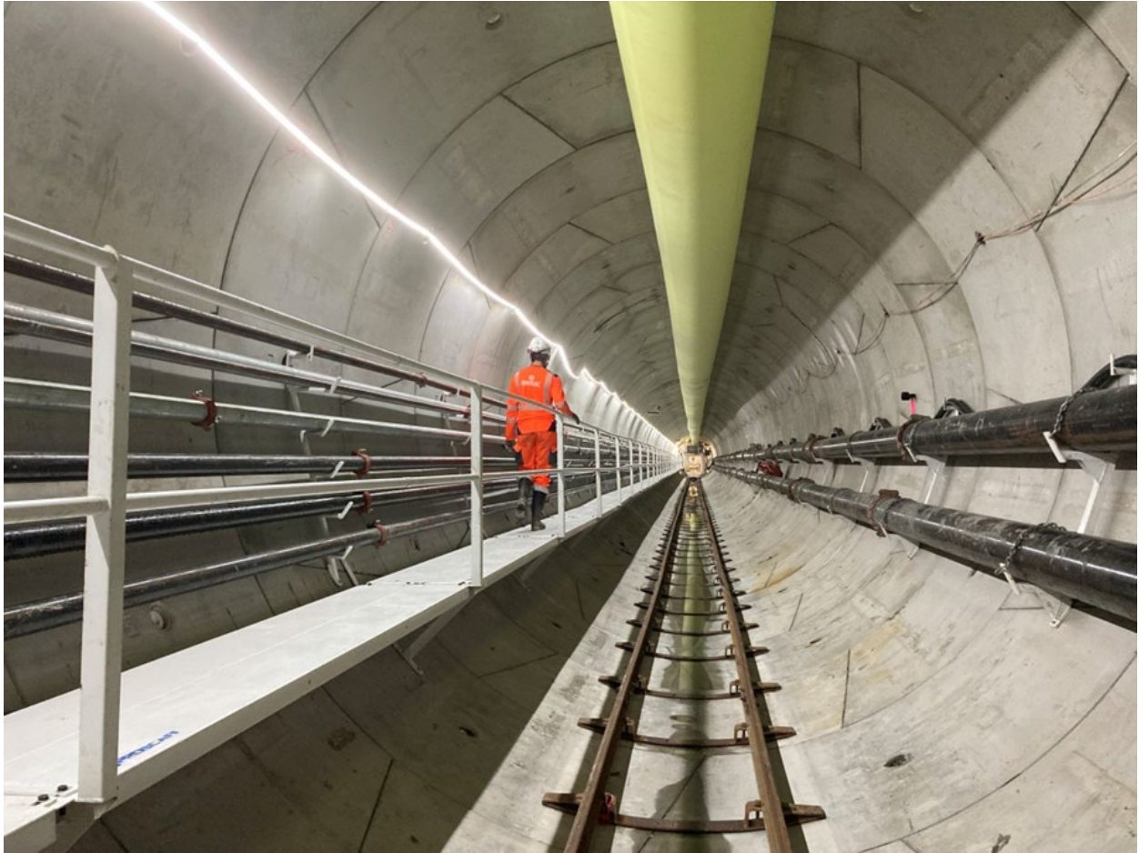
Graphic 8 Example of a TBM Tunnel Showing Pre-cast Lining Segments. Upon completion, temporary utilities and infrastructure would be removed to enable haul truck access.
