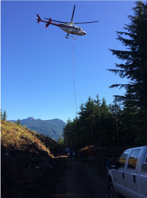
Figure 6. Example of Helicopter Stringing
