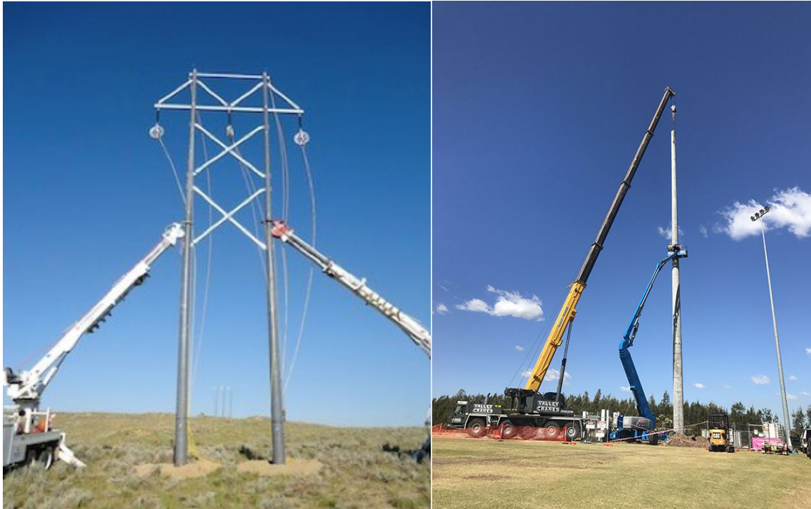
Figure 5. Example of Cranes Assembling Transmission Towers
