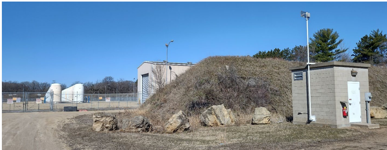
Figure 10: Current Instrumentation Building Near the ISFSI
