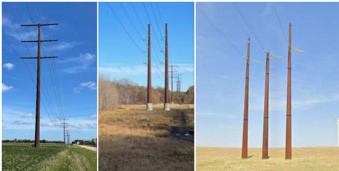
Typical Double-Circuit Structures
