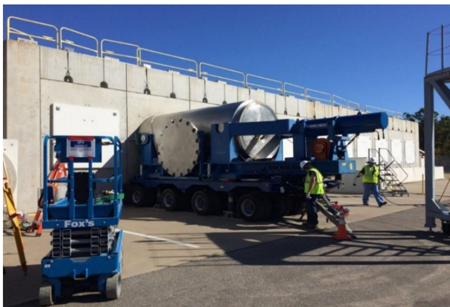
Figure 3: Placement of Canisters in Horizontal Concrete Overpack
