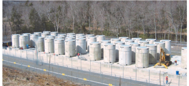
Loaded spent fuel storage casks are in place on storage pad at the Haddam Neck Plant in Meriden, CT. (Courtesy: Connecticut Yankee)
