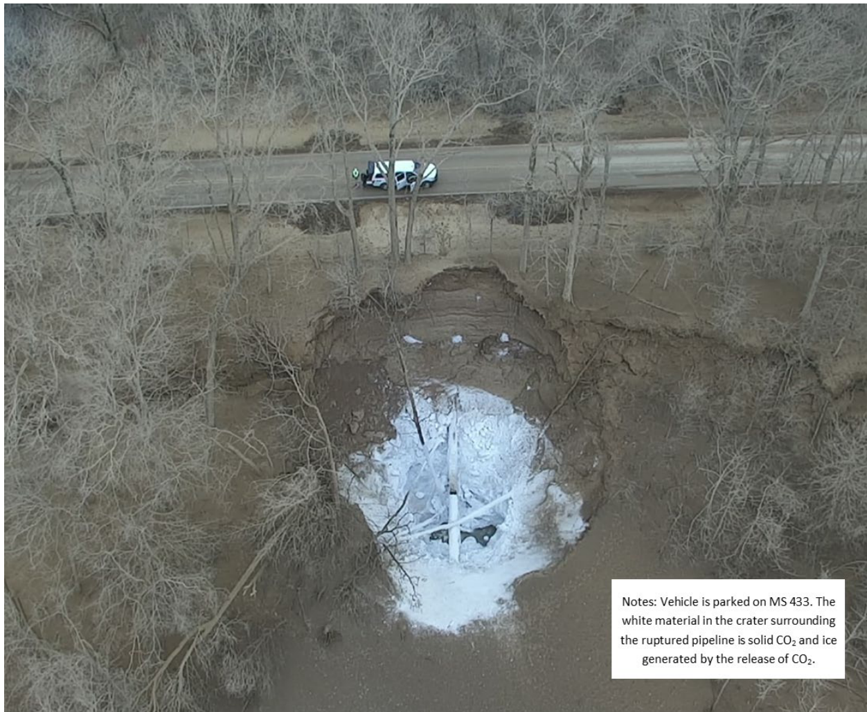
Figure 8-1 Photo of Pipeline Rupture Site near Satartia, Mississippi
