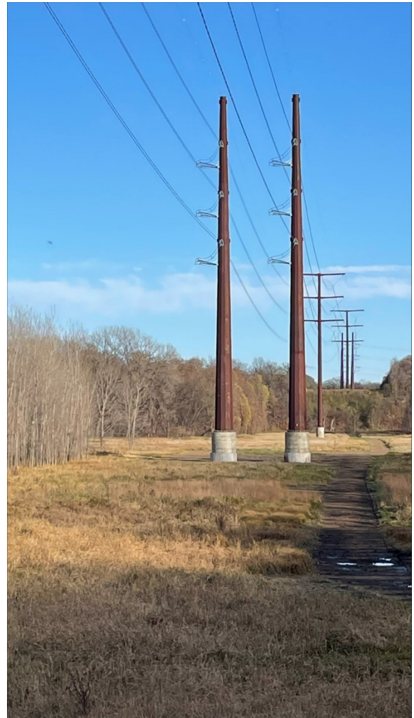
Two-pole structures for angles and dead-ends
