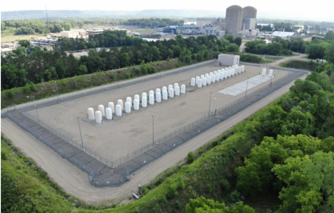
Photo: Prairie Island Plant ISFSI with 50 TN-40/40HT Dry Fuel Storage (DFS) systems stored on 3 concrete pads. Photo taken by Nuclear Innovation Team drone, July 2023.
