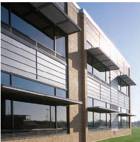
Protect all glass areas exposed in summer with deep recesses, overhangs, or other devices to minimize heat gain.
