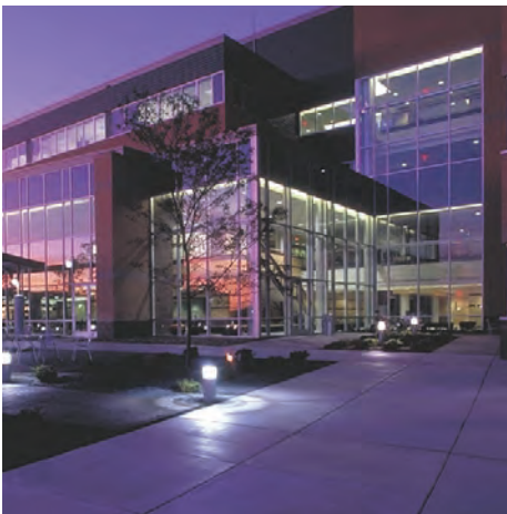
Prominent building entries that face the street.
