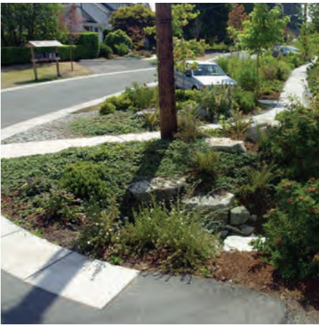
Proper stormwater treatment
