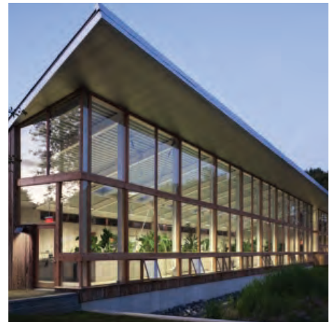
Sustainable building design reduces energy use
