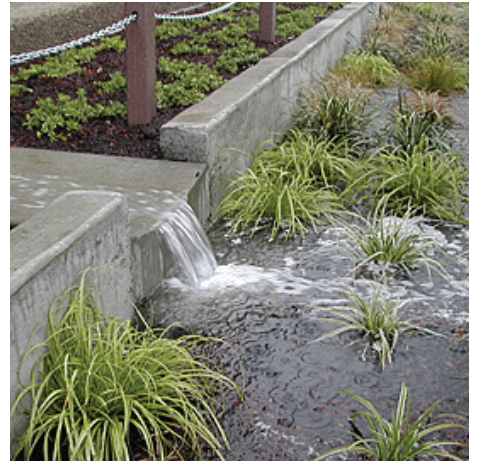
Water from roof tops and impervious surfaces should be used for irrigation of landscaping.
