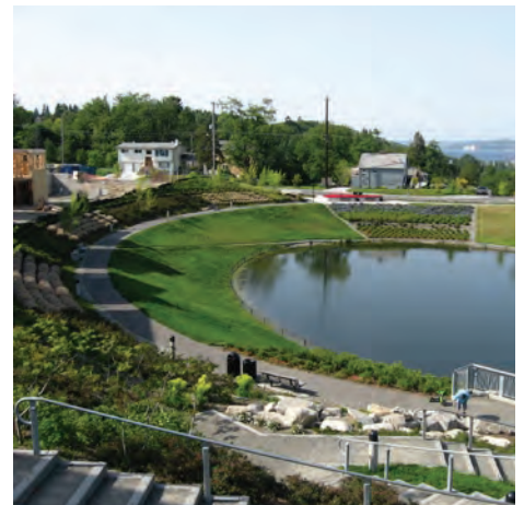
Stormwater ponds should be integrated with the open space system and treated as an amenity.
