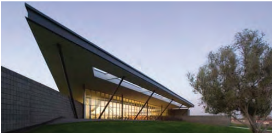
Orient buildings on the site to take advantage of the site's microclimate, solar, daylighting, natural ventilation and energy flows.
