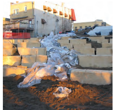
Soil erosion protection
