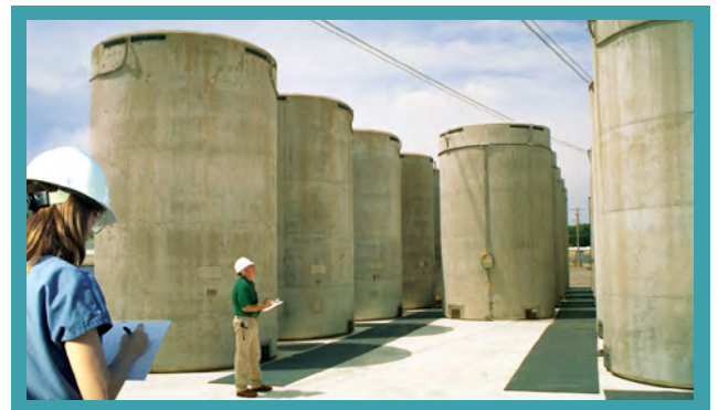
After the cooling period, nuclear energy facilities store used fuel safely on-site in steel and concrete vaults.
