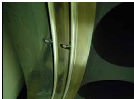
RPV O-FLEX™ Seals with installation clips
