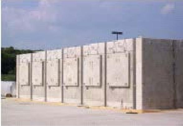
Currently, the only horizontal system available is the TN NUHOMS (Nuclear Horizontal Modular System) designed, licensed and manufactured by Orano, Inc. The system is used at several nuclear power plants throughout the United States as well as at several foreign reactors.
