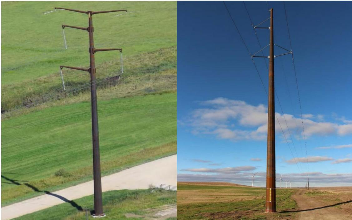
For the portions of the transmission project located within county road ROW (approximately 7.8 miles, for Route A and 11.2 miles for Route B, DCW proposes to use a braced post design with shorter spans between structures in order for the alignment to be located within the road ROW. Road ROW widths along these segments range from approximately 66 to 100 feet in width for Route A and approximately 66 to 150 feet for Route B.
