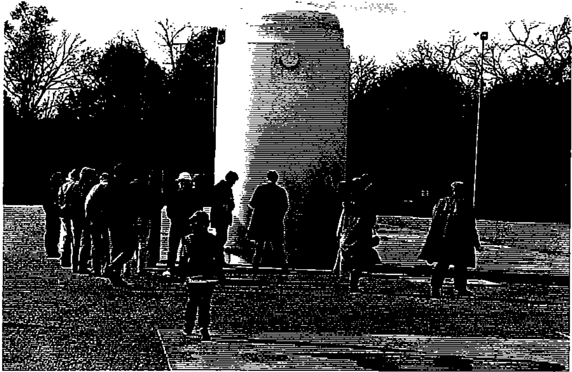
Task Force Tour of Prairie Island Nuclear Waste Storage Facility, October 28, 1995.
