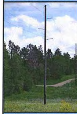
Typical 115 kV Wood Single Circuit Structure
