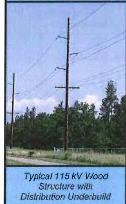
Typical 115 kV Wood Single Circuit Structure
