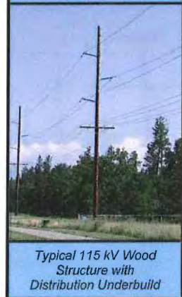
Typical 115 kV Wood Single Circuit Structure
