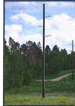
Typical 115 kV Wood Single Circuit Structure
