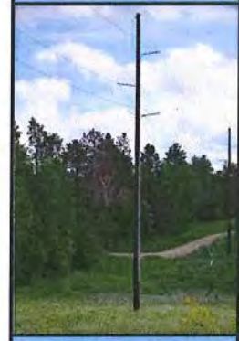
Typical 115 kV Wood Single Circuit Structure
