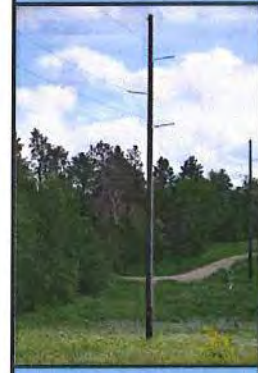
Typical 115 kV Wood Single Circuit Structure
