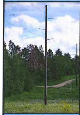
Typical 115 kV Wood Single Circuit Structure
