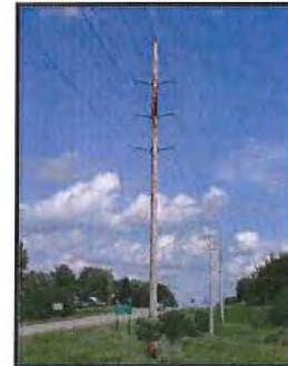
Typical 115 kV Wood Double Circuit Structure
