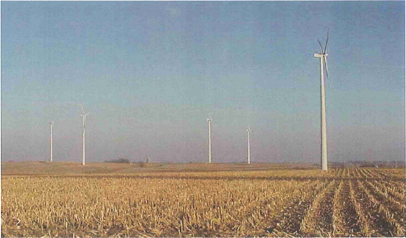
Top of Iowa project – developed and built by Midwest Renewable Energy Partners, a company partly owned by EBF at time of development
