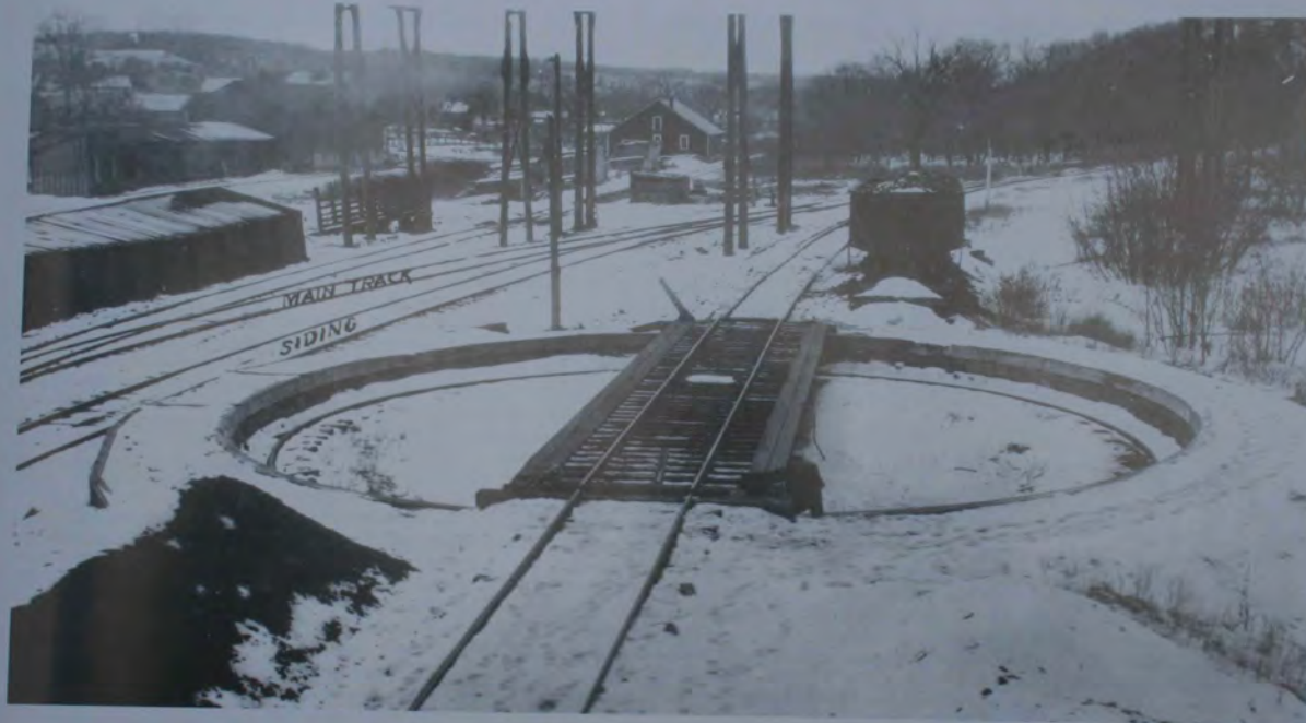
This bird's eye view of the turntable at Taylors Falls was captured on film on March 4, 1925. The photographer climbed the ladder on the engine house to get this excellent view of the railroad facilities looking south. Notice the car of coal spotted along side the turntable lead track. The engine's tender would be positioned next to the coal car, and then the engine house watchman would shovel what must have seemed like several tons of coal into the tender. The coal track was slightly elevated, but not nearly enough, and the poor watchman probably didn't shovel more than he absolutely had to. The building on the left is the stockyard shelter shed. Cattle loading was generally done on the far left siding, but an additional cattle loading chute more accessible can be seen on the left. Farther to the left are some warehouses and a local coal facility. A large lumberyard is far off in the center along side the long spur that was originally extended for the St. Croix Lumber Company. In the foreground is a pile of cinders and ashes from various locomotives that tied up here for a layover. Iron Horse Central Museum collection
