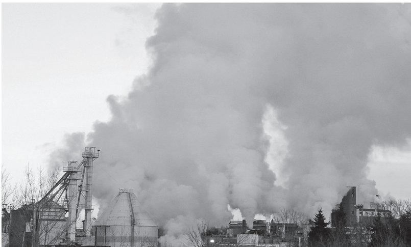
Engineers say the warm air and steam currently vented by Rock-Tenn has the potential to be captured to heat commercial buildings on University Avenue and the Central Corridor stations.
