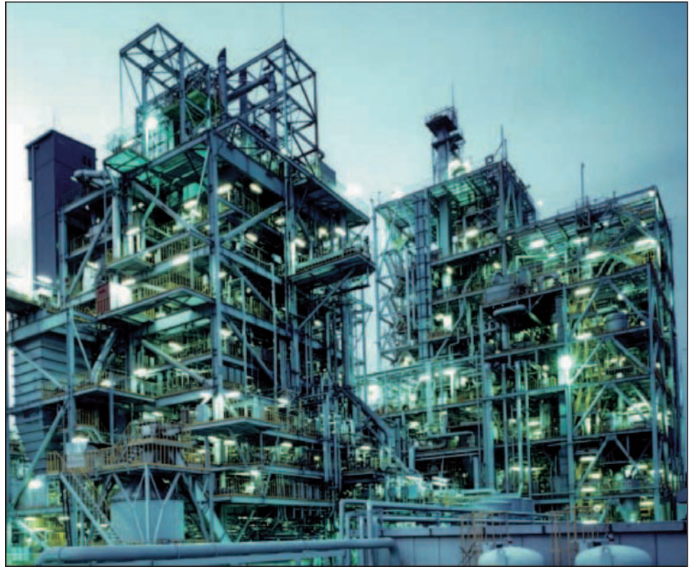
Nakoso 200 tpd pilot plant. Design included a 12.5 MW gas turbine (but no bottoming steam turbine) and a developmental hot gas clean-up system. Oxidizing air for the air blown gasifier was extracted from the turbine. Pilot plant testing ended in 1995.
