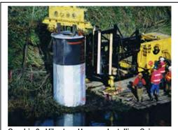
Graphic 2: Vibratory Hammer Installing Caisson
