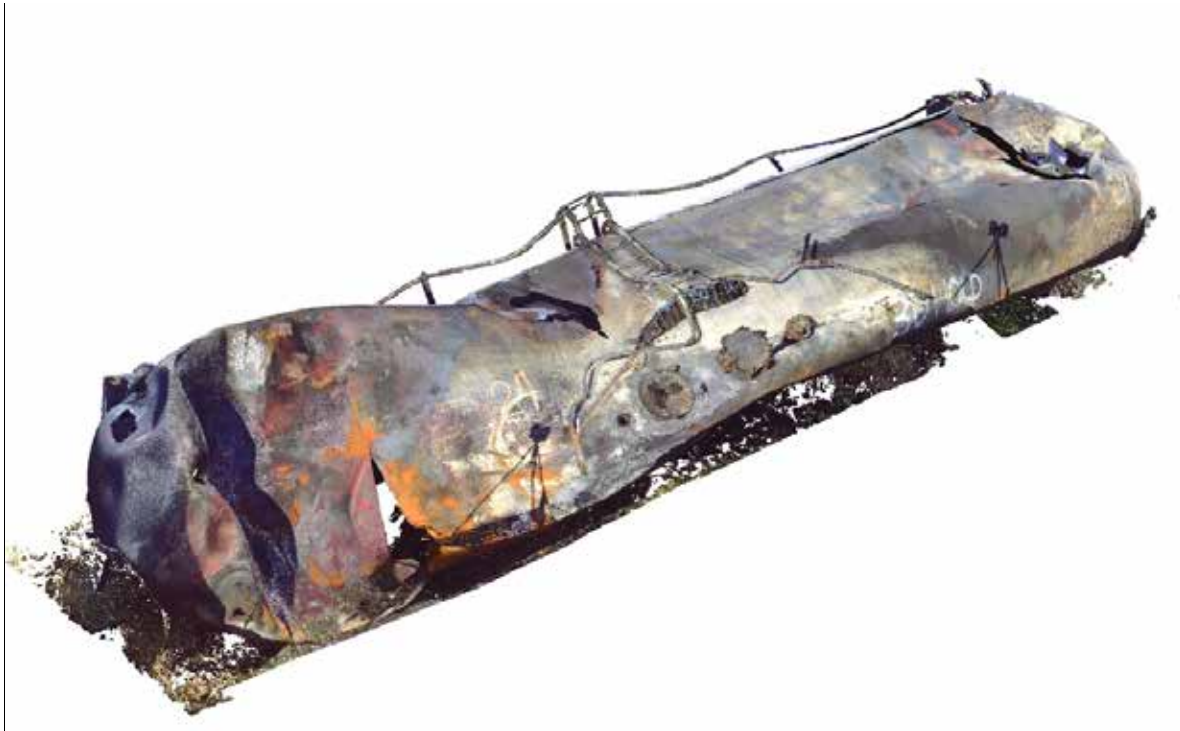
Photo 16. 3D laser scan of badly deformed tank
