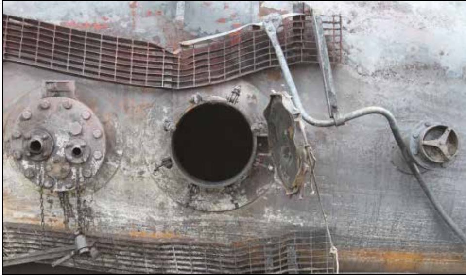
Photo 23. Manway cover and opening
