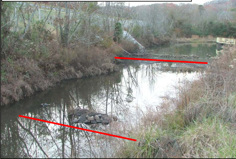
Fig. 11 Breached Check Dams
